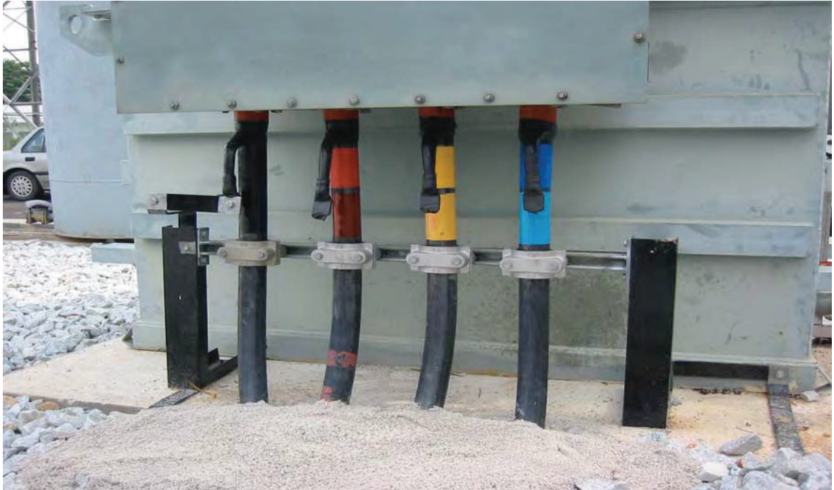
BATU TIGA 132/33 kV SUBSTATION ( Earthing Transformer )
