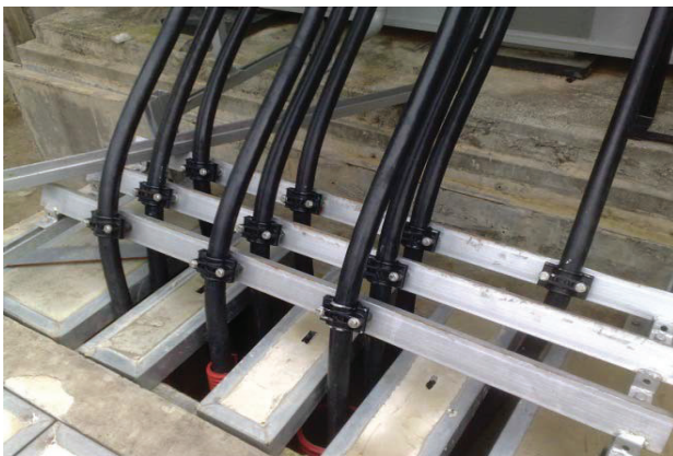
Cable cleats installed for 11 kV Power Cables
