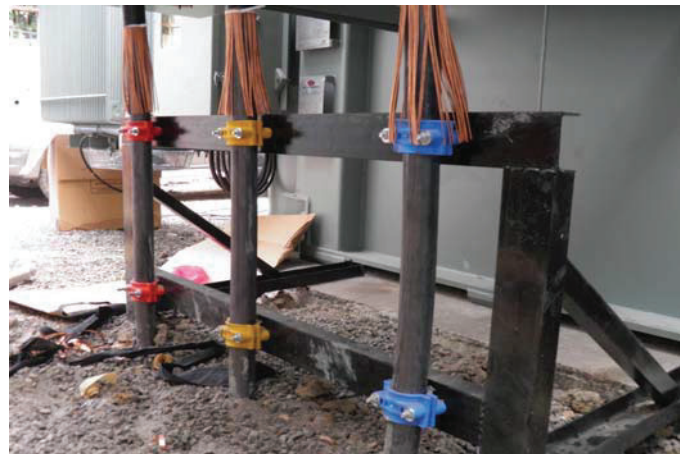
Coloured Cable cleats installed at the LV side
