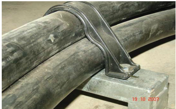
Non-Metallic Trefoil Cable Cleats installed at Ampang 275 / 132 kV substation.
