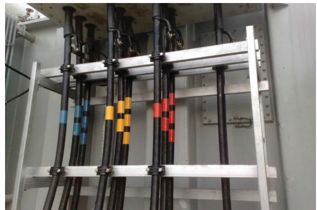
Cable cleats installed for 275 kV power Cables
