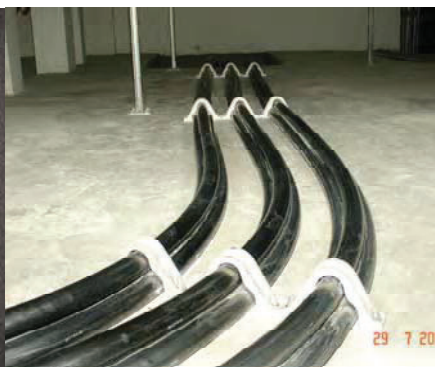
Aluminium trefoil cable cleats at Kota Damansara 132, 33 and 11 kV Substation.
