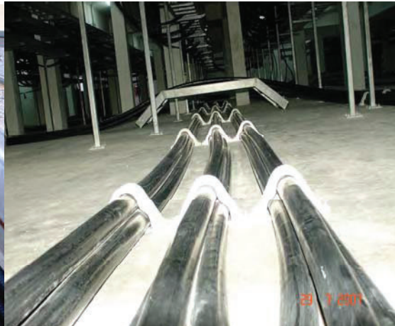
33 kV Aluminium Power Cables.
