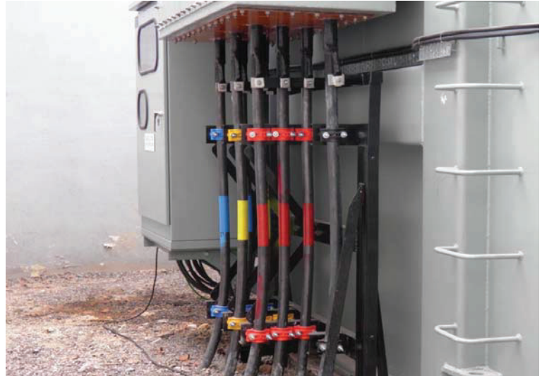
Coloured Cable Cleat used for easy identification of phases
