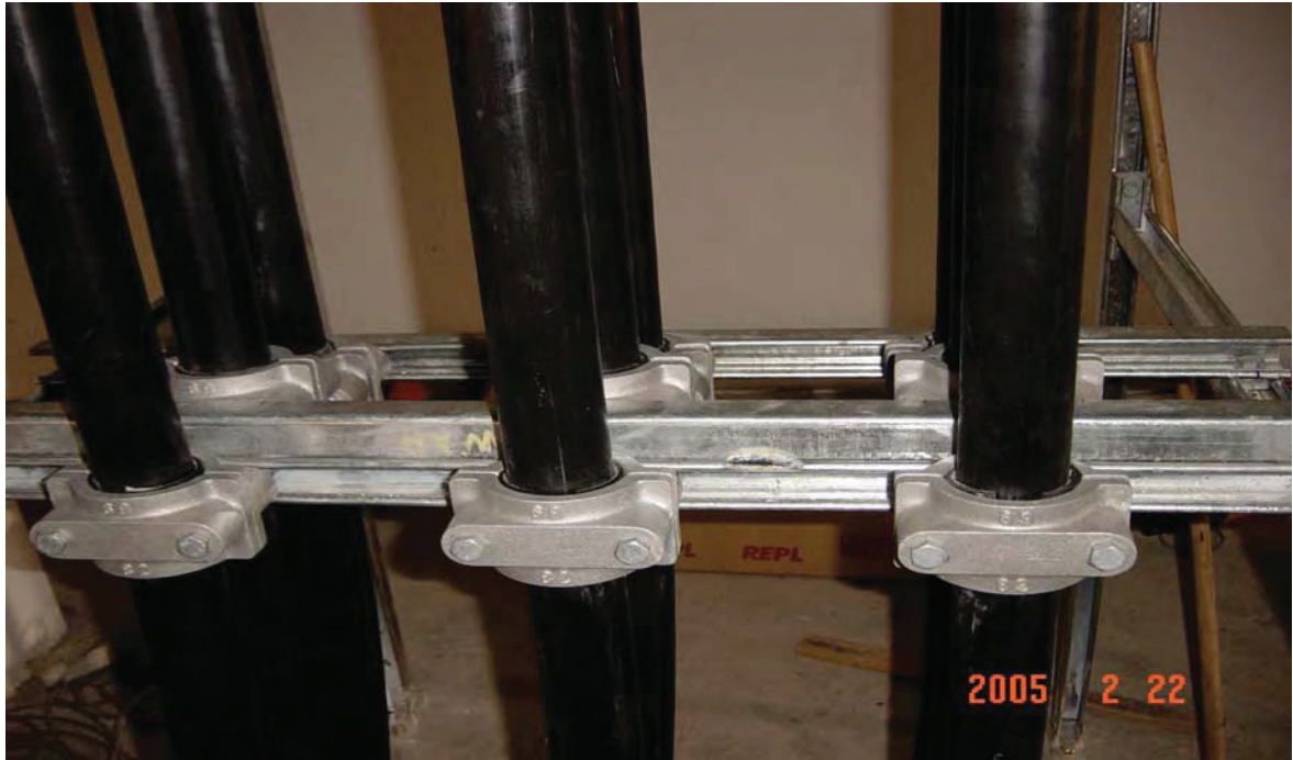
Close up view of Cable Cleat ( XLPE power cable 630mmsq
