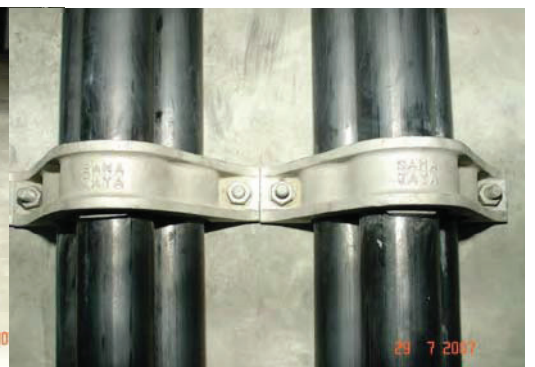
Aluminium trefoil cable cleats (fire proof ) installed at Pengkalan 132 kV S/S.
