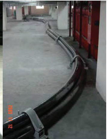
275kV Power Cables
