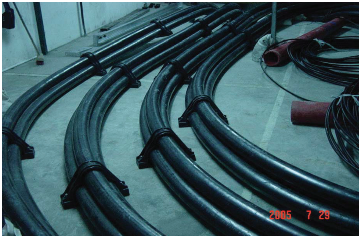
Non-Metallic Trefoil Cable Cleats installed at cable cellar at Silibin 132 kV Substation.
