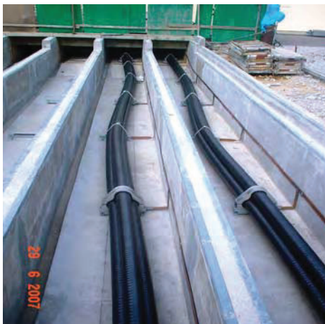
275 kV Power Cables
