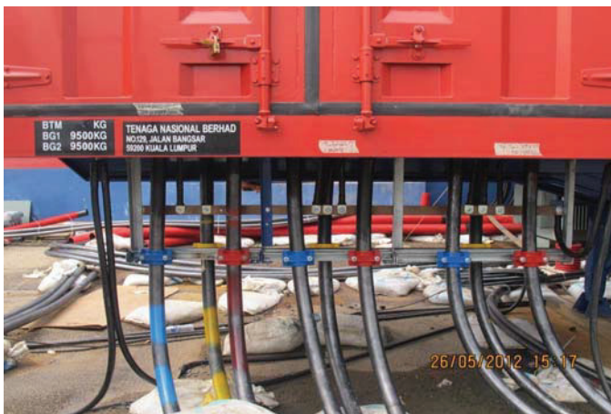
Coloured Cable cleats installed in a mobile substation
