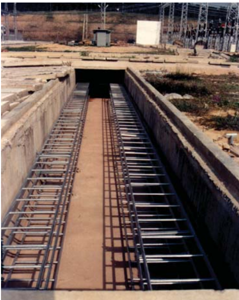
Pasir Panjang 132kV Substation.
