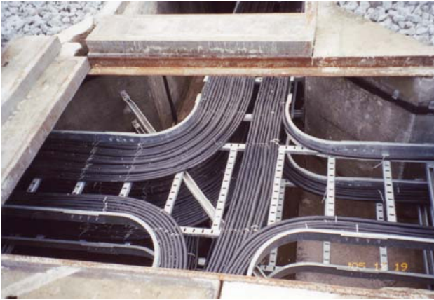
Pengkalan Industry 132/33/11 kV Substation, Perak
