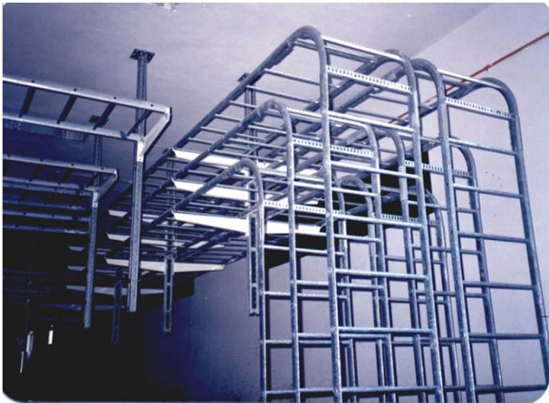
Serdang 275/132 kV Substation
