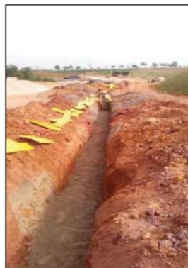
Laying of fine Sand (covering the gas pipe)
