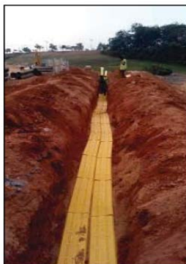
Laying of Protection Cover for gas pipe
