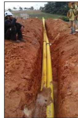
Laying of Gas Pipe
