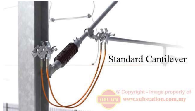
Cantilever Section using Double Short Rail Earth
