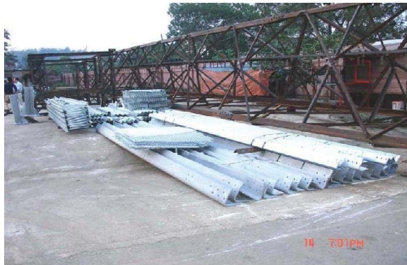
Fabrication of equipment steel structure support
