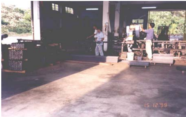
Fabrication of Steel Member in Progress
