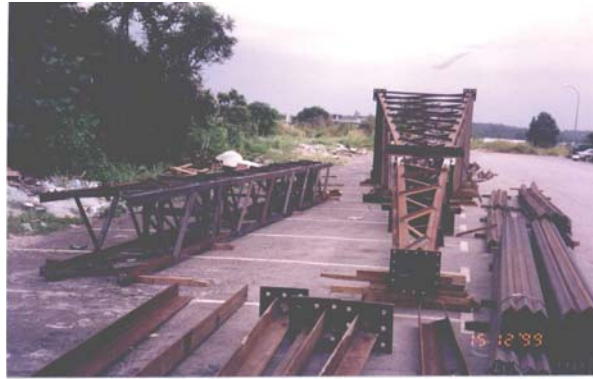
Front View of 132kV Substation Gantry Tower And Gantry Beam
