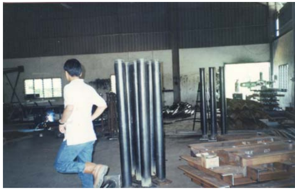
Anchor bolts with welded plates
