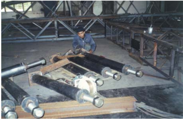
Another view of anchor bolts
