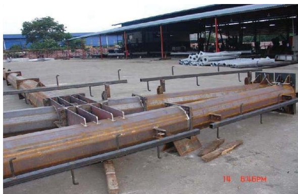
Fabrication of different types of Towers and Beams
