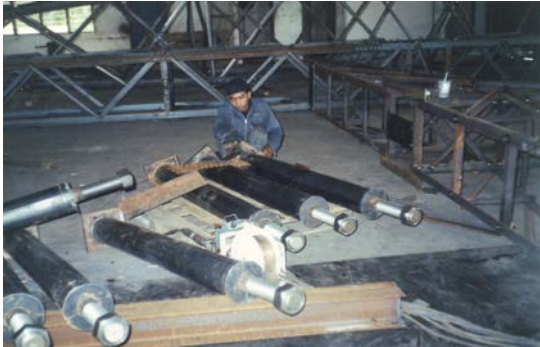
Another view of anchor bolts
