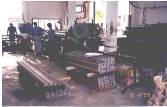
Punching of Holes at Steel Member in Progress
