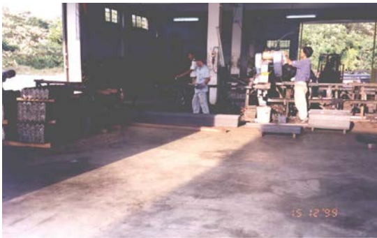
Fabrication of Steel Member in Progress
