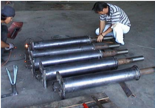
Anchor Bolts and Sleeve Fabrications
