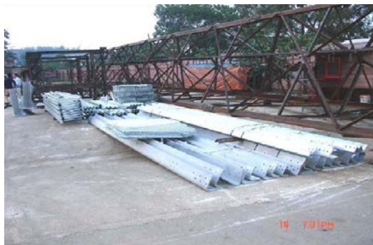
Fabrication of equipment steel structure support
