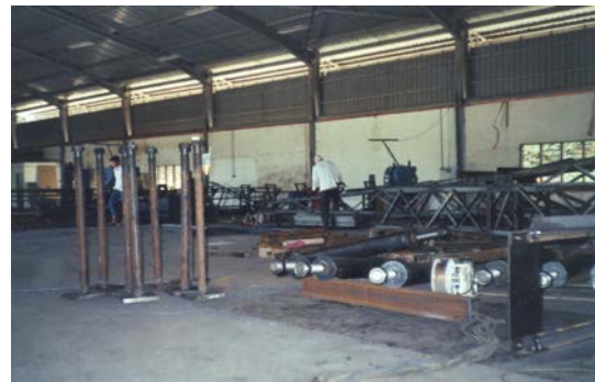
Anchor Bolts with Foundation Embedded Plate
