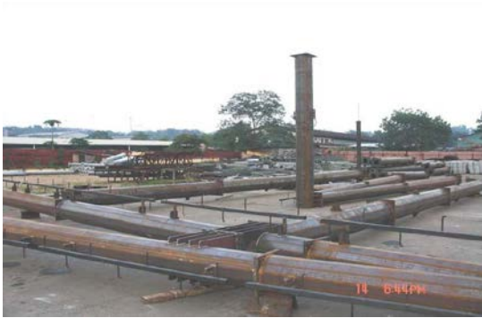
Assembled Towers and Beams for customer inspection
