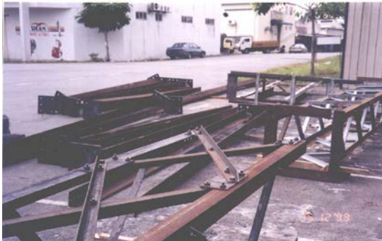
Assembled Steel for Customer Inspection
