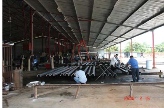
Fabrication of different types of Towers and Beams
