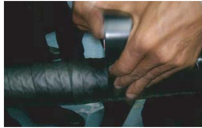
Scotch No.23 Insulating Tape being applied for cable insulation.
