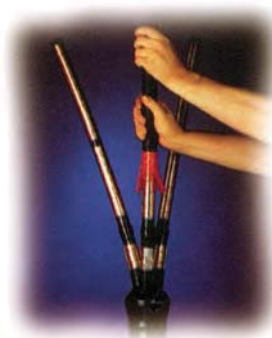
Slide on the Re-jacketing Sleeve.
