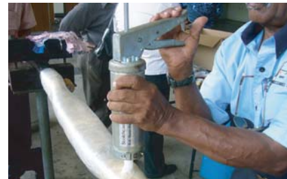
Resin being injected into the joint with the Scotchcast E-4 Resin Pressure Gun.
