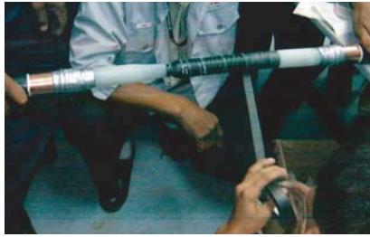
Scotch No.13 Semi-conducting Tape being taped over the crimp connectors.
